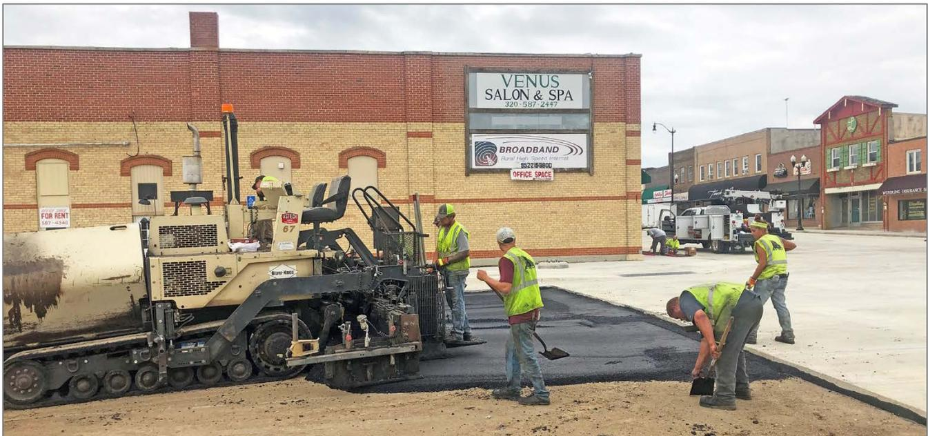
Photo above: paving the asphalt tie-in to the new concrete on Main Street at 1<sup>st</sup> Avenue South.
