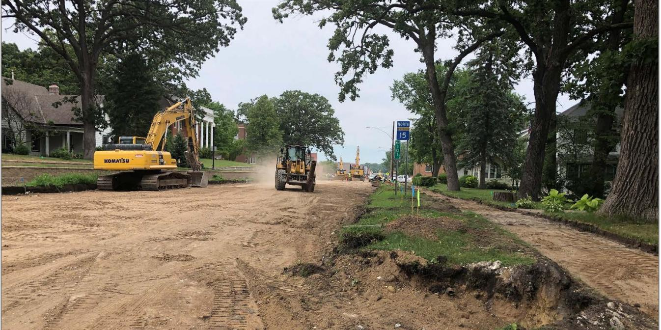
Photo above: (looking north) removing old pavement and sidewalk south of 4<sup>th</sup> Avenue South.
